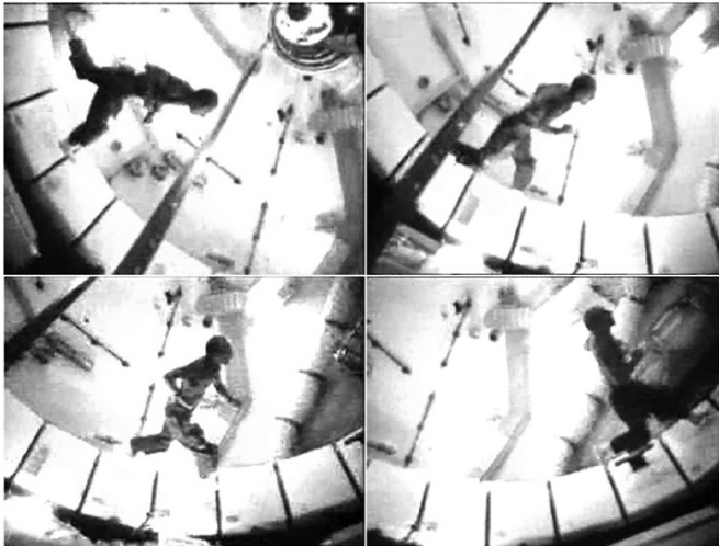
Figure 8-12. The diameter of the Skylab workshop was wide enough for the astronauts to generate the right amount of centrifugal force that allowed them to run along the rim of the cylindrical module. This activity provided them with both artificial gravity and exercise. Photo courtesy of NASA.
