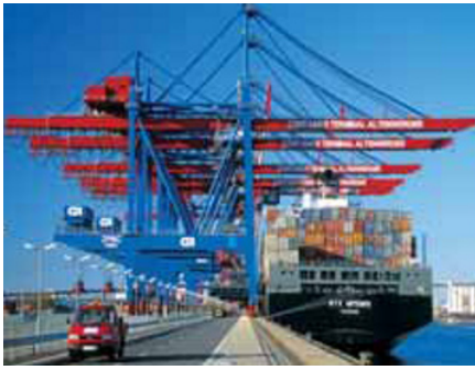
(a) Quay cranes (here: dual-trolley crane) serving a vessel (courtesy of HHLA).
