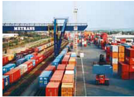
(b) Waiting trains under a gantry crane; a reachstacker on the right (courtesy of HHLA).
