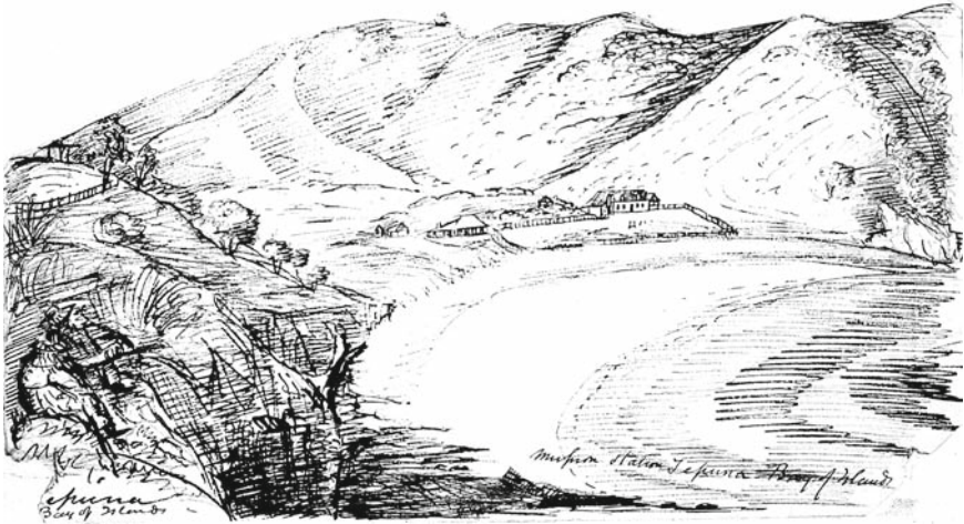
Figure 4.12. Te Puna Mission Station, looking toward the east, c. 1839–1841 (Artist Richard Taylor, 1805–1873. Alexander Turnbull Library, Wellington, New Zealand. E-296-q-160–1)
