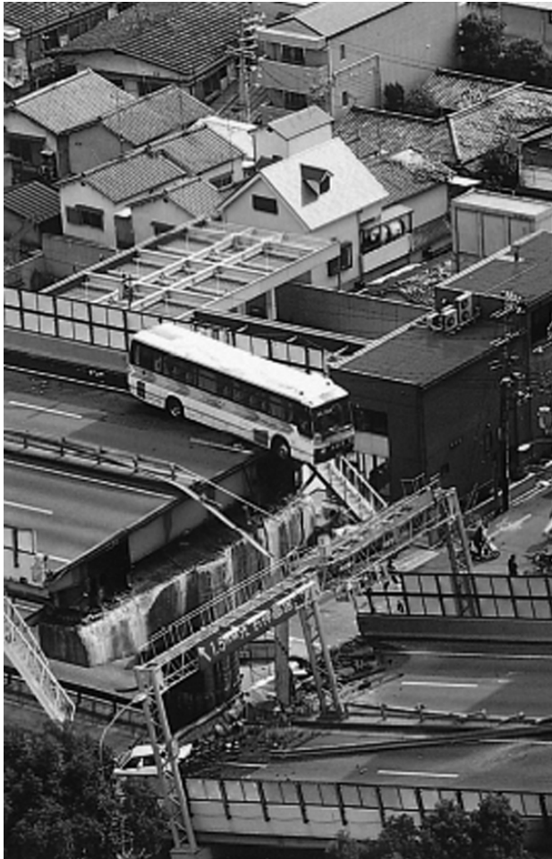
Fig. 7 The earthquake of Kobe in 1995 damaged many infrastructure lines (Photo: © dpa-Bildarchiv)
