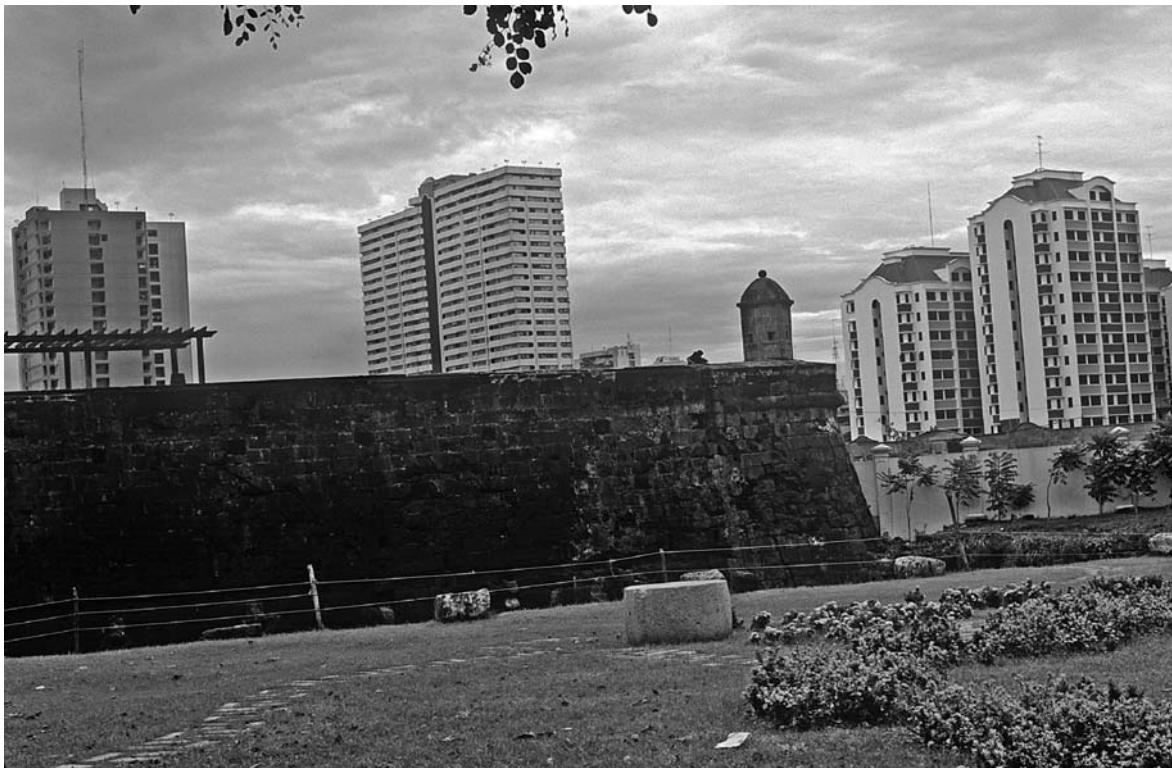
Fig. 8 Restored fortifications of Intramuros with modern Manila in the background (photograph by the author, 1995)
