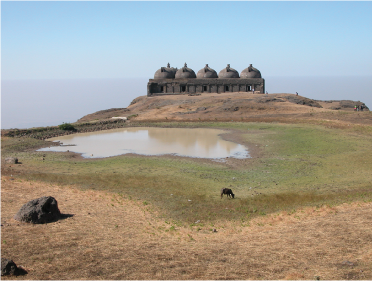
Fig. 3 Water collection reservoir at Naulakha Kothar. (Photo by author, January 2005)
