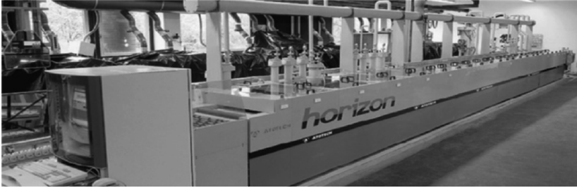
Fig. 9.14. Production line for application of immersion tin (Source: Atotech)
