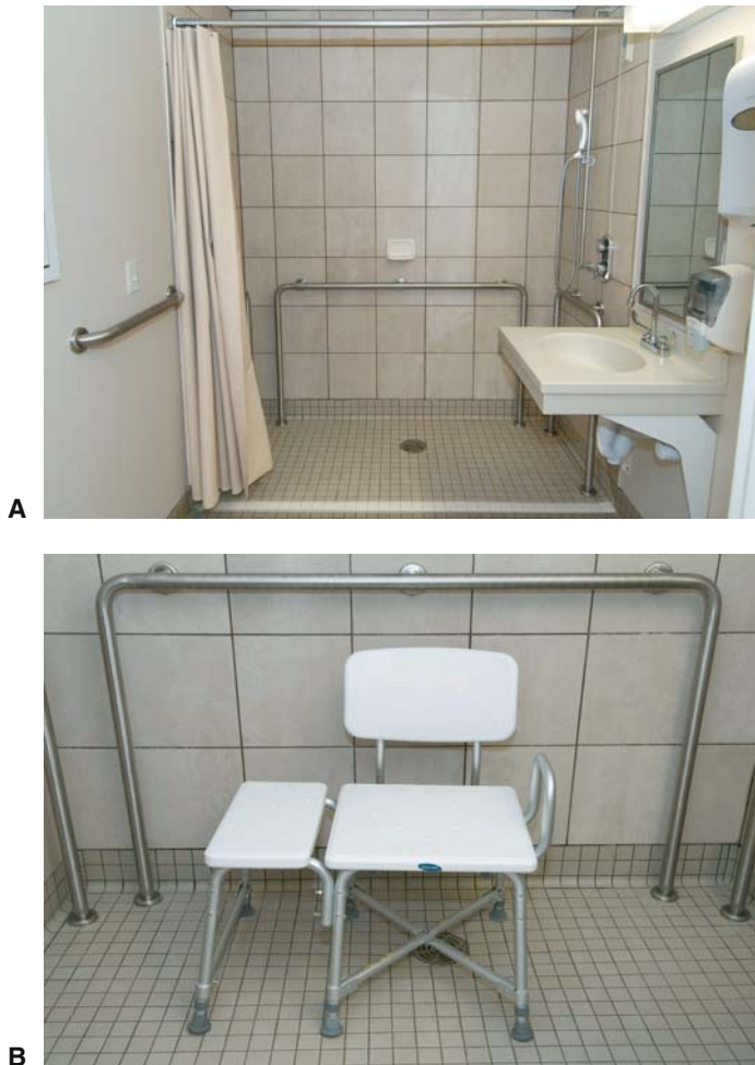
FIGURE 6-12. (A) Large shower room with unobstructed access to shower. (Courtesy of Bariatric and Metabolic Institute, Cleveland Clinic Foundation, Cleveland, OH). (B) Shower chair (Courtesy of Sizewise Rentals, www.sizewise.net .)
