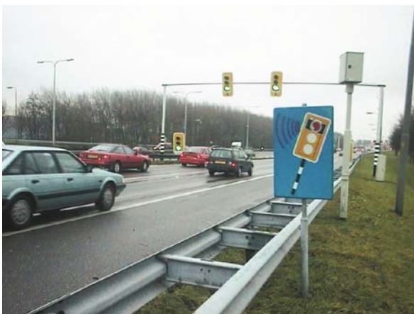
Freeway Traffic Management and Control, Figure 7 Ramp metering at the freeway A13 in Delft, The Netherlands. One car may pass per green phase. To prevent red-light running the control is enforced
