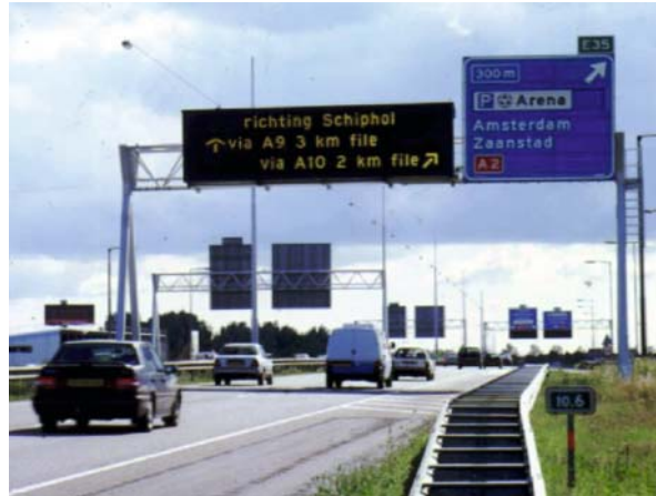
Freeway Traffic Management and Control, Figure 9 A route guidance system in The Netherlands showing traffic jams on alternative routes to Schiphol Airport (Photo courtesy of Peek Traffic B.V.)
