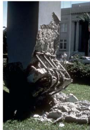
Earthquake Damage: Detection and Early Warning in Man-Made Structures, Figure 6 Imperial County Services (ICS) building: a view (towards north); b photographs of damage: columns F1 and F2 at the ground floor; and c column F1
