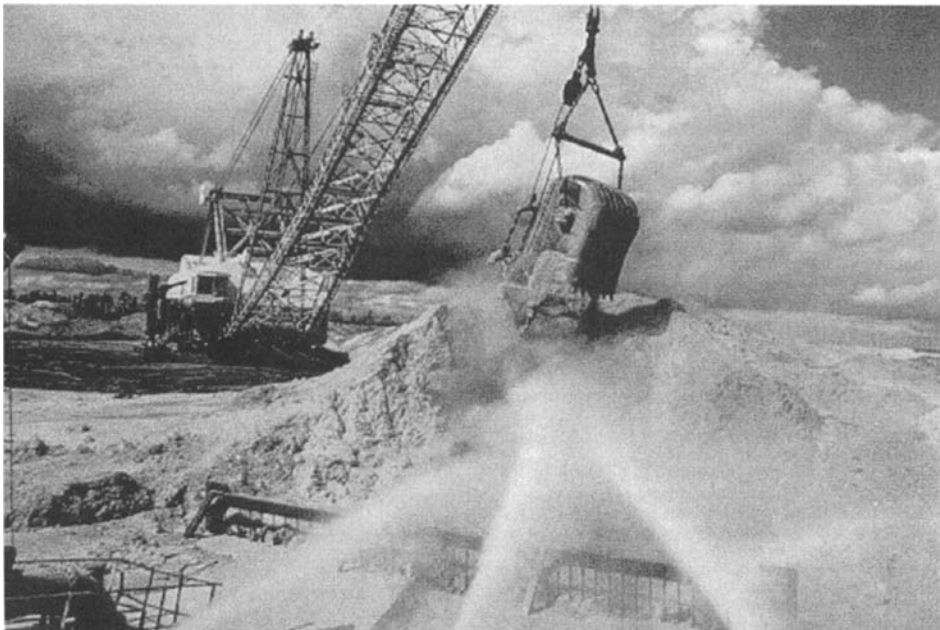
Fig. 23.4. Gunning phosphate rock in a Florida mine.
