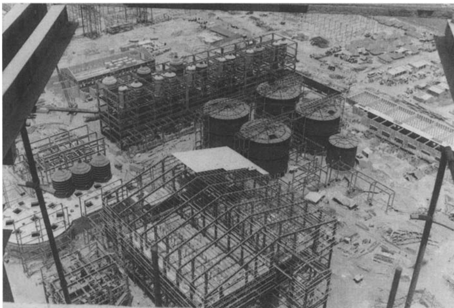
Fig. 23.10. Oswal phosphoric acid plant during construction—May 1999—in Paradeep, Orissa State, India.
