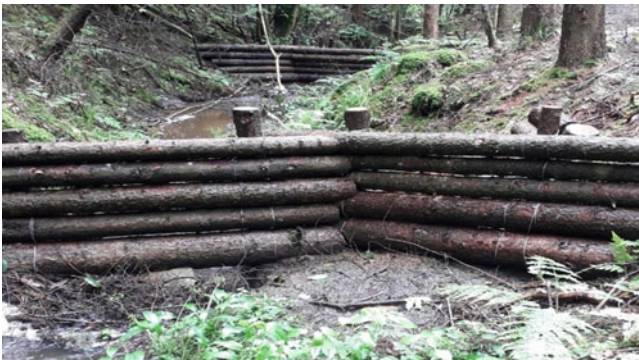
Fig. 9 Leaky barriers structure applied in the torrential river, after Hankin et al. [19]
