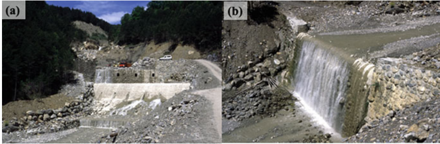
Fig. 7 (a) Construction of new check dams in the lower stretch of the Arás ravine (Upper Gállego basin), following the collapse of most of check dams during the extreme flood of August 1996; (b) New check dam in the lower course of the Arás ravine (Upper Gállego basin). It was constructed after the collapse of most of check dams during the extreme flood of August 1996 (Photos JM. García-Ruiz)
