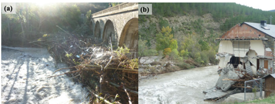
Fig. 3 Some effects of the 19–21 October flood 2012 in the Central Spanish Pyrenees. (a) The bridge over the Aragón River at Jaca, dammed by a large mass of trees carried by the floodwaters; (b) A family house destroyed after the October flood (Aragón River) (Photos E. Nadal-Romero)
