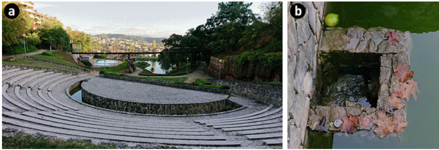
Fig. 5 View of the Amphitheatre in the foreground, with a small water retention volume (a), and the reduced outlet connecting to the settling ponds (b)
