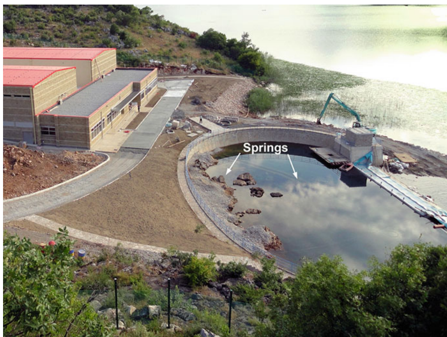
Fig. 9 Water source “Bolje Sestre” during construction (photo by Milan Radulović)
