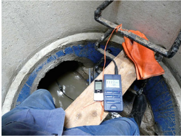
Fig. 13 Measuring device in a manhole
