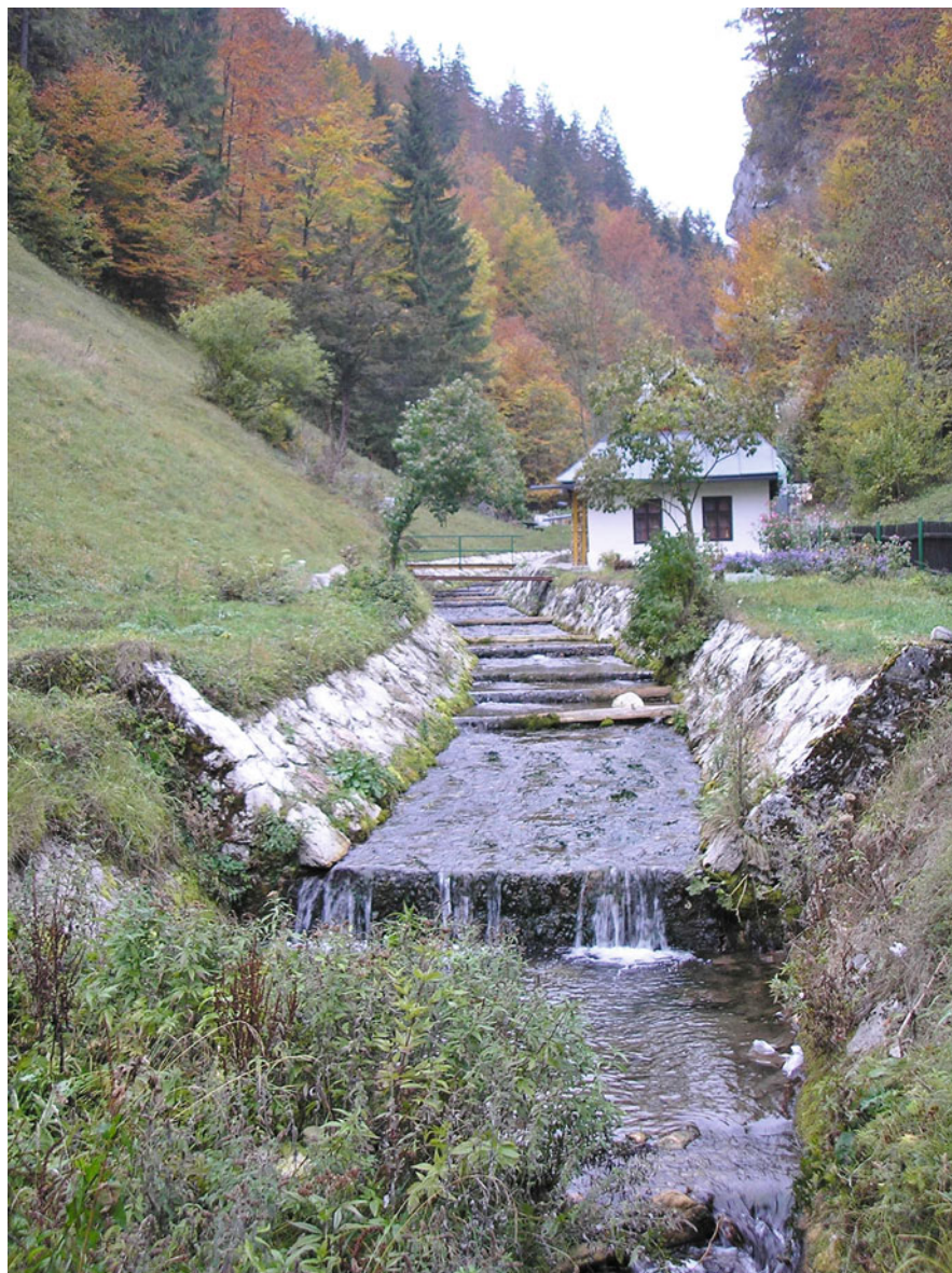
Fig. 5 Longitudinal reinforcement by pavement stone, the stone weir, and system of wooden sills in the oldest torrent control – Jelenec in Hornojelenecká Valley from 1926 to 1927 (photo M. Jakubis)
