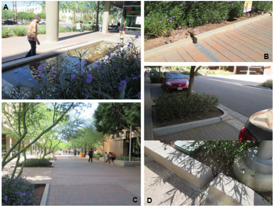
Fig. 5 (a) Water features can harvest rainfall, making water visible and celebrating its importance in an arid climate. (b) Grated curb cuts convey storm water from pavement into planting areas. (c) Porous pavers and permeable pavement at the pedestrian walkway allow infiltration and reduce off-site runoff. (d) Standard curb cuts open up planting areas to receive storm water flow [20]
