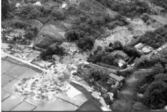
Fig. 1. Mudflow type slope failure during the 2003 earthquake in Japan
