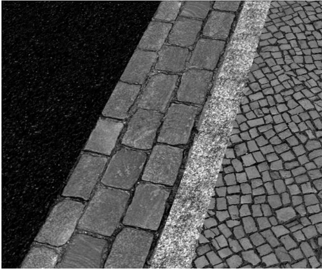
Fig. 8. Examples of kerbs along the border lines of streets and sidewalks
