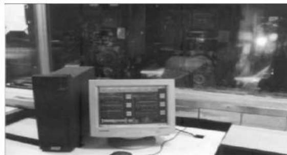
Figure 2. OPPRESS system in service to HSM, Tata Steel, India
