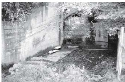
Fig. 2. The mine entrance in 2000.
