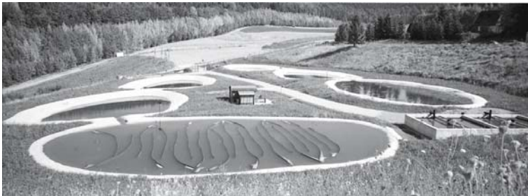
Fig. 7. Photograph of the constructed wetland at Poehla, Autumn 2004.
