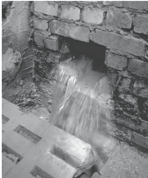
Fig. 4. Discharge point at the dewatering adit (MP1).
