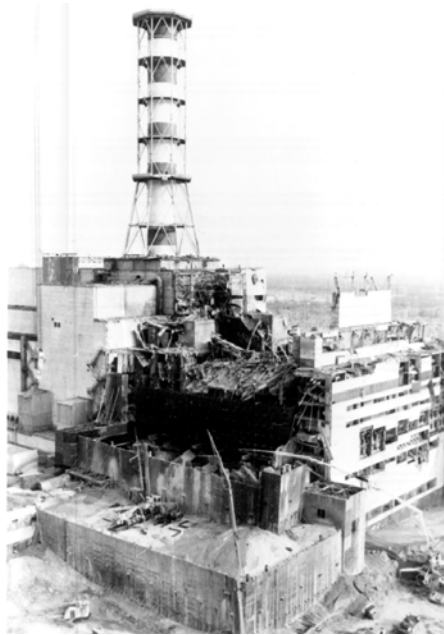
Figure 1.5. Sarcophagus construction, early September 1986: construction of the northern cascade wall.
