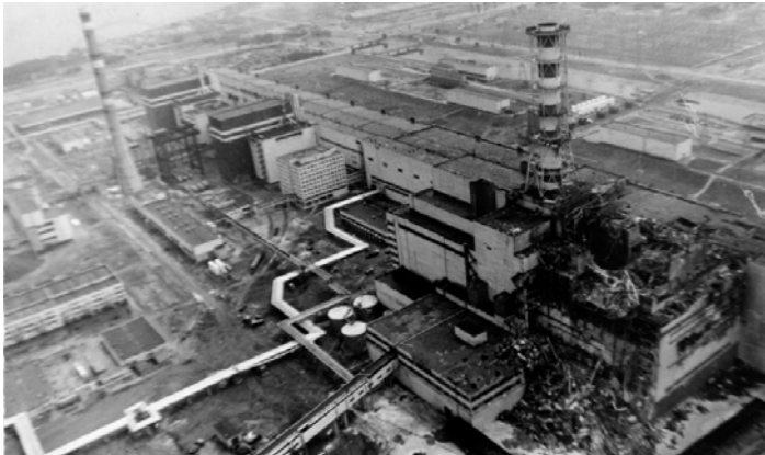
Figure 1.1. The destroyed Unit 4 reactor building at the Chernobyl Nuclear Power Plant (NPP). The edge of the Cooling Pond can be seen top left.
