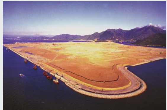
Fig. TB2.10.3. View of the Hong Kong International Airport construction site during 1995 (© K. Bartlett, Pacific Century Publishers Limited)
