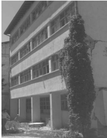
Fig. 3. Digital photo of the damaged schoolhouse obtained by KODAK DCS 200 and plumb lines used as scale information
