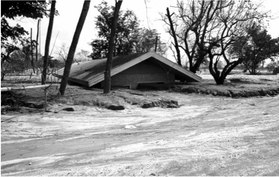
Figure 8.14. Burial of house and trees downstream of Mount Pinatubo, Philippines, due to river bed aggradation resulting primarily from repeated, relatively small hyperconcentrated flows that spread out on the alluvial fan after the stream channel was filled with sediment.
