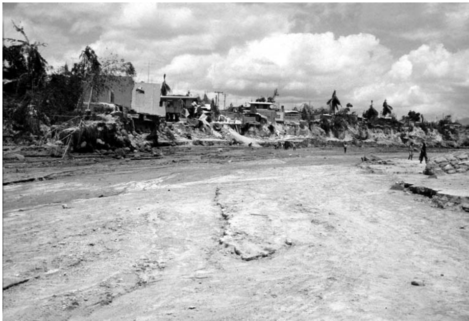
Figure 8.15. Destruction of buildings along a river bank downstream from Mount Pinatubo, Philippines, caused by lateral erosion of channel banks by hyperconcentrated flows.
