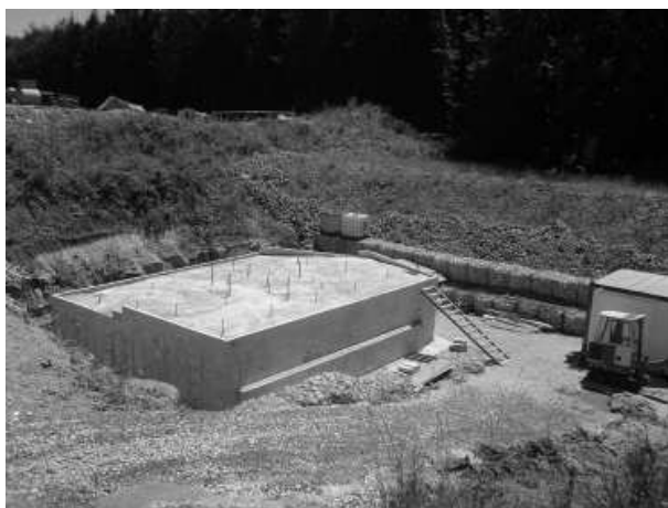
Fig. 5.10. Completely encapsulated field block; direction of view: south-east.
