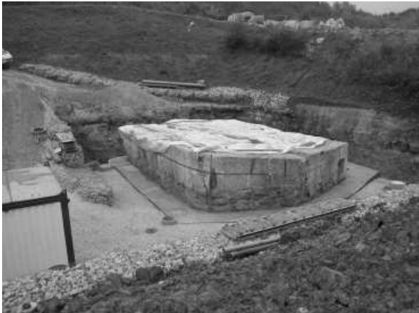
Fig. 5.8. Unsealed field block with concrete ring foundation; direction of view: north-east.
