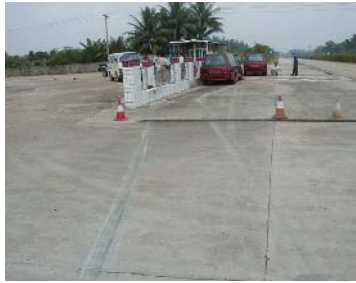
Fig. 1. The photo of the accident scene
