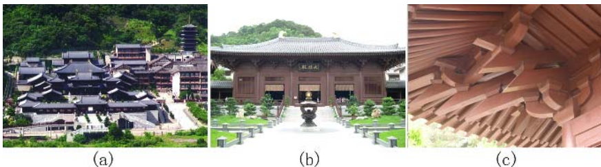
Fig. 1. (a) The timber-frame building complex. (b) A hall in the complex. (c) A set of Toukung.
