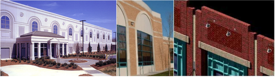
Fig. 1. Example walls that are not easily represented in current parametric models. They each show mixes of materials and properties that will not be reflected in costs or energy assessments.
