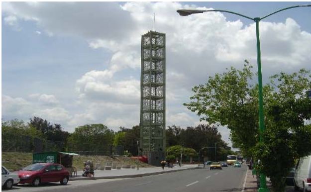
Fig. 1. The camera is placed on top of this 28-meter tower
