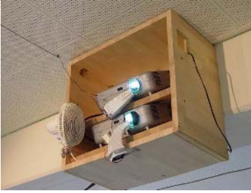
Fig. 2. Left: The shuttered stereo projection system. Right: The virtual model of the exhibit at the CeBit 2006 in Hannover.
