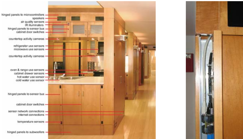
Fig. 2. Sensors are located throughout the cabinetry in a consistent way in every room of the apartment. Some sensor locations are indicated here (left). All of the observational sensing is built directly into the cabinetry. Although the sensors are ubiquitous, they become part of the design aesthetic (small black windows). Pilot volunteers have expressed that they are easy to forget. The cabinetry has been designed with channels for the sensor bus, making it easy to distribute sensors throughout the environment. The channels hinge open, allowing easy access for maintenance and sensor additions/upgrades (right). Adding a sensor simply requires adding a splitter in a channel (circled) and plugging in the device.
