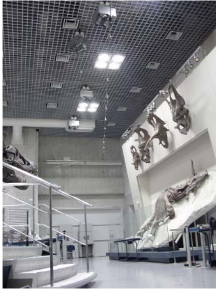
Fig. 12. Installed Transmitters for Dynamic Positioning
