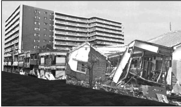
Fig. 8. Kobe City after the 1995 Earthquake (By Stefan Lisowski)
