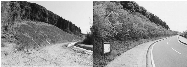
Photo 3. An example of formation of an evergreen and deciduous broadleaved tree community established using the TGM method (Case Study C). Left: After 4 months, Right: After 6 years.
