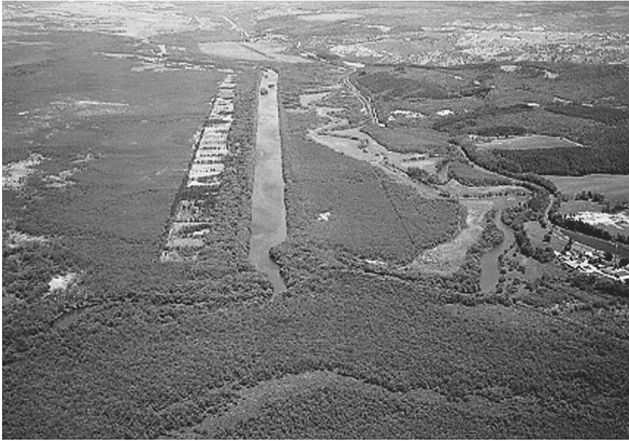
Figure 8. The restoration project of meandering river. River flows from up to bottom of the picture. The meandering section (right side) will be connected to the main channel.
