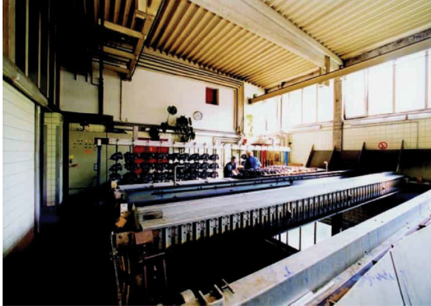
Figure 7.4 The anodising plant at Eloxieranstalt A. Heuberger GmbH
