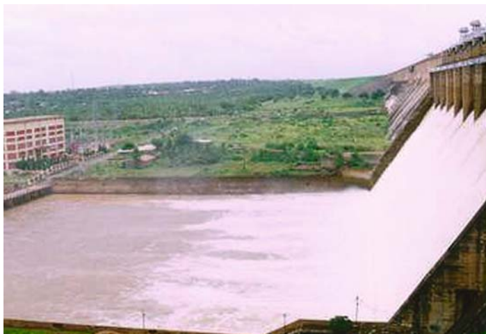
Figure 10. A view of Ghatprabha dam (Hidkal dam)
