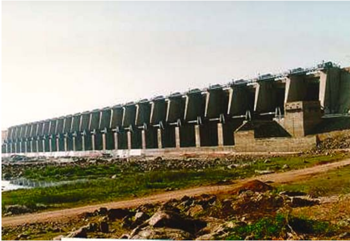
Figure 6. A view of Narayanpur dam
