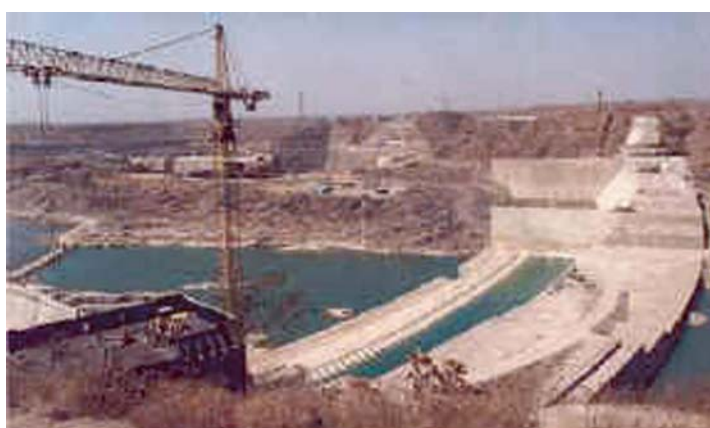
Figure 9. Indira Sagar Project (Under Construction)
