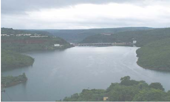
Figure 8. A view of the Srisailem dam and reservoir
