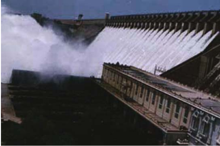
Figure 9. A view of Nagarjunasagar dam
