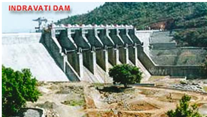
Figure 15. A view of Indravati project
