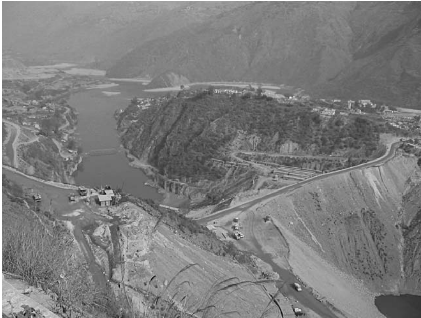
Figure 15. A view of Tehri dam (under construction)
