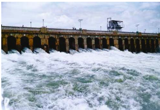
Figure 3. A view of KRS dam
