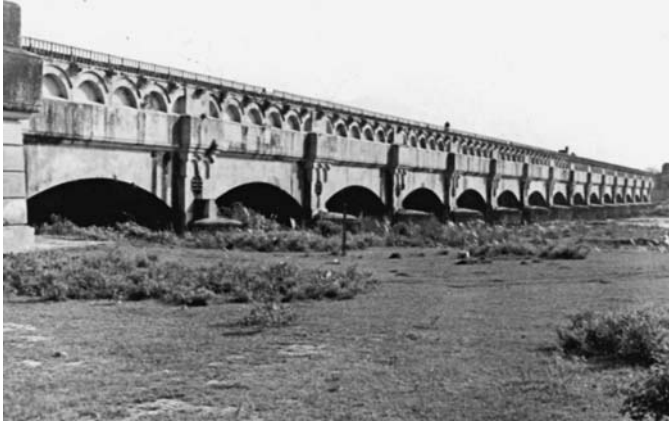
Figure 13. Old Solani aqueduct of the Upper Ganga Canal near Roorkee
