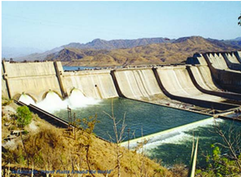
Figure 7. Main Sardar Sarovar dam (Under construction)
