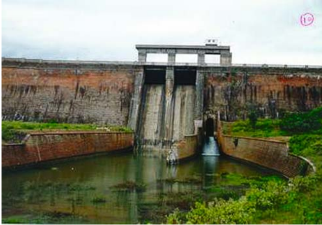
Figure 5. Nugu dam in Cauvery basin
