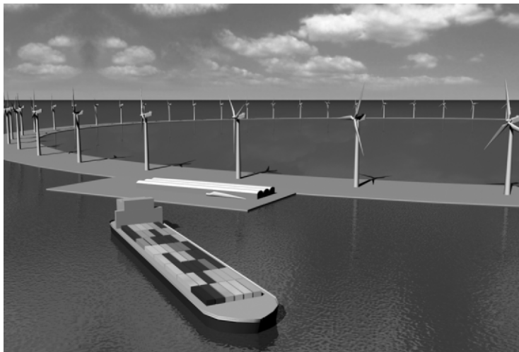
Figure 1. Artist view of an offshore wind farm on a ring dike for better accessibility of wind turbines for maintenance and repair. [Please see this figure in the color section at p. 311]
