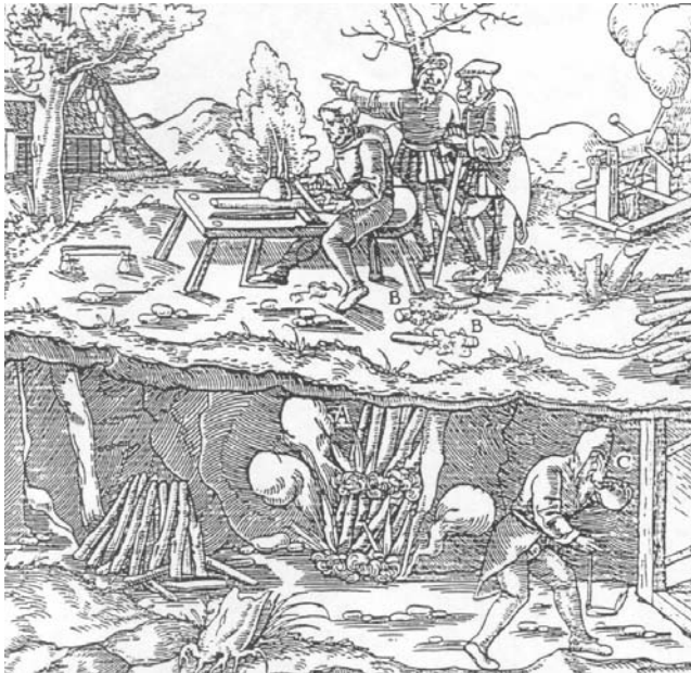
Figure 18-4. Underground fire setting (Agricola, 1978)
