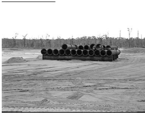
Figure 20-16. The sand deposit at Bige. The pipes are used to conduct the sand-water mixture from the river to the deposit. This is a very familiar sight to Hamburgians, since contaminated dredge from harbour basins and the shipping channel is disposed of using the same technique.
