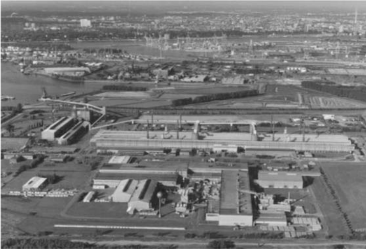
Figure 13-1. HAW aerial view.
