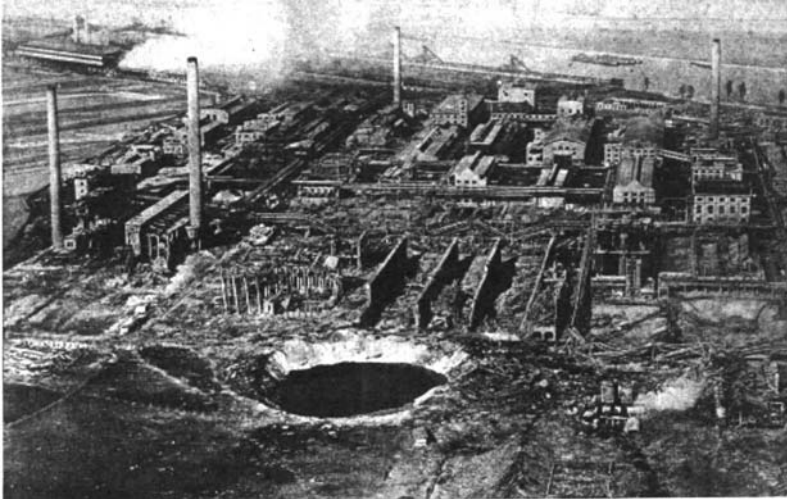
Figure 17-3. Explosion accident site in Oppau 1921
