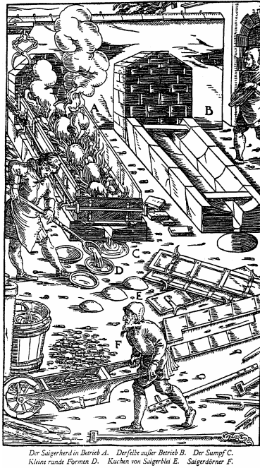
Figure 18-18. The PbAg-Cu “Saiger process” in “Saiger furnaces” (Agricola, 1978)
