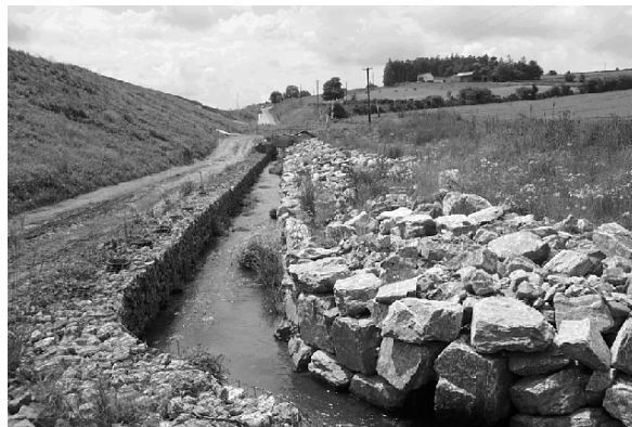
Figure 1. Rock armouring, gabions and stream. (Dolan & Whelan)
