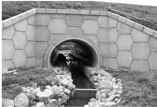
Figure 2. Arched culvert with mammal ledge (Dolan & Whelan)
