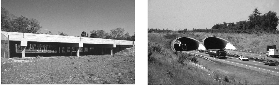
Figure 1. Wildlife-crossing structures that provide animals a safe passage across transport corridors: A wildlife underpass ( left ) that links Florida panther habitat across State Road 29 in Big Cypress National Preserve, US, and wildlife overpass ‘Woeste Hoeve’ ( right ), constructed to help ungulates across highway A50 in The Netherlands.
