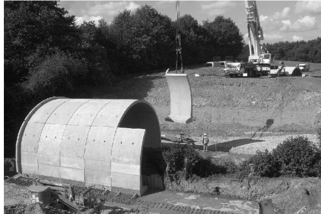
Figure 6. Culverted road, United Kingdom (photograph E.O'Brien courtesy of ABM Construction)
