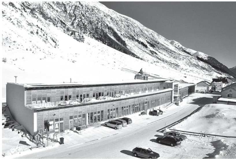
Figure 2. Aerial view of the Alpinarium (Source: Alpinarium Dokumentation GmbH, 2002).
