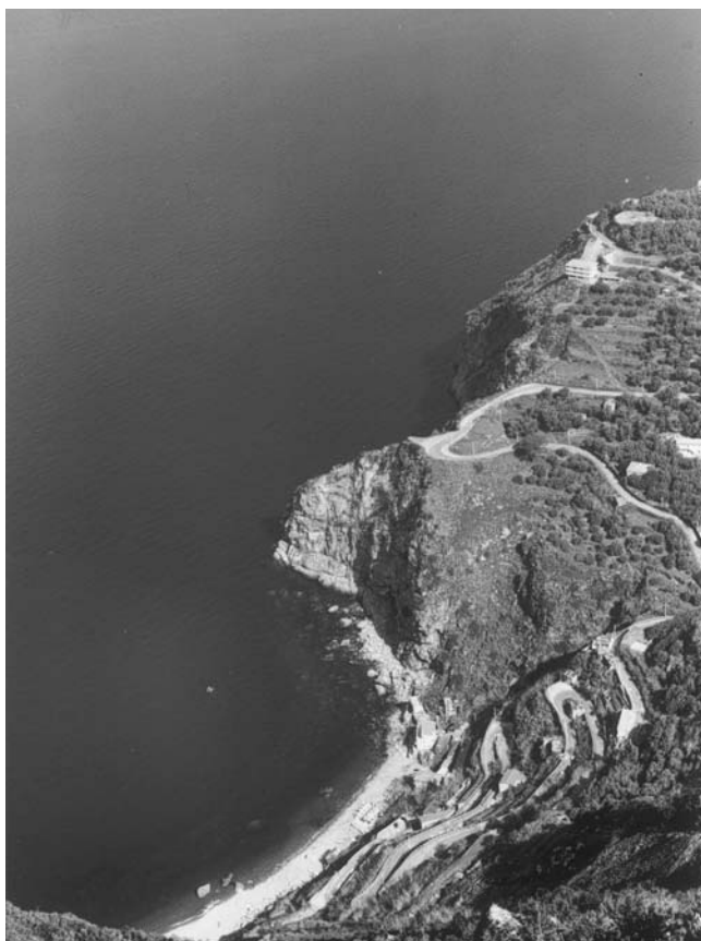
Figure T8 The active fault scarp near Palmi (Calabria, Italy) (photo E722, April 1996).
