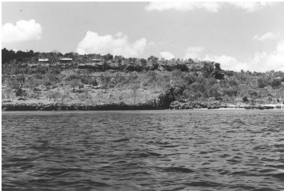
Figure T7 The surface of Late Pleistocene raised marine terraces has been displaced by a recent fault near Kupang, West Timor, Indonesia (photo B266, August 1988).
