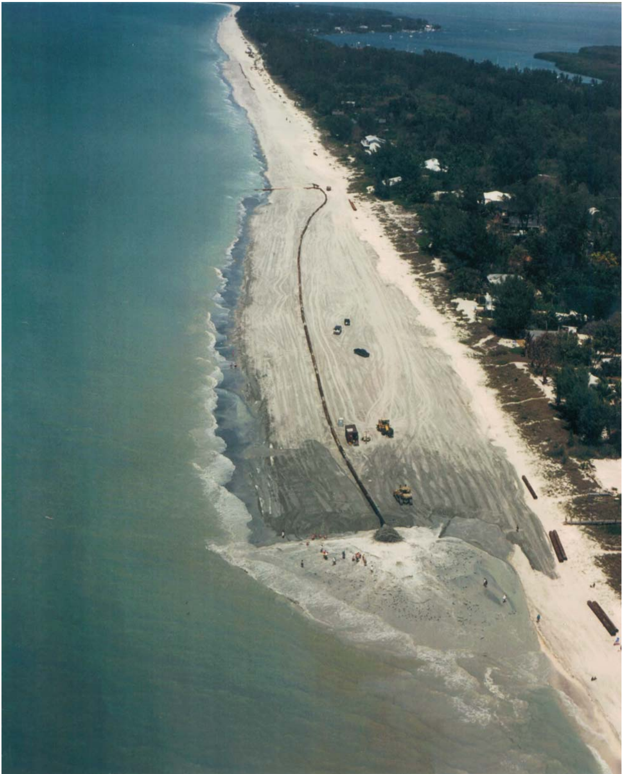
Figure B30 Restoration of Captiva Beach in 1996 on Sanibel Island, southwestern Florida, showing beach-quality sand pumped from offshore via a submerged pipeline to the shore. The sand–water slurry debauches from the pipe end (lower center foreground) to form an alluvial fan that builds up along the shore. Shell hunters often congregate about the proximal part of the sediment fan hoping to find collector's specimens. Shore birds search the distal portions of the fan for crustaceans brought up from the seafloor in the offshore borrow area. Road graders and bulldozers redistribute the pumped sediment into the beachfill design shape that often incorporates overfill that will be sacrificed to the littoral system as the beach equilibrates to the ambient wave climate. The beachfill is sometimes initially somewhat darker than the native beach sand, as shown here, due to a small percentage of organic content. Organic matter in the fill bleaches out within a few weeks and the native-colored sands imperceptibly grade into the fill material. Pipe extensions lie at the foot of the foredunes (photo, lower right) and mark the approximate position of the back berm (photo: Courtesy of Coastal Planning and Engineering, Inc., Boca Raton, FL).
