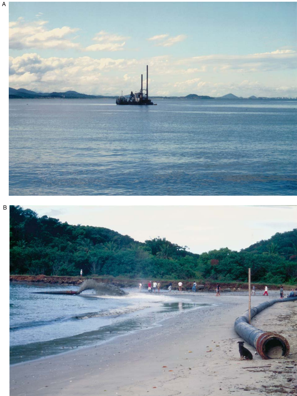
Figure B28 Small-scale beach renourishment at Alegre Beach, Santa Catarina, Brazil. Local erosion of a beach on the downdrift side of an inlet required sand renourishment for shore protection, recreation, and marine fisheries (beach launching sites for local fisherman). (A) The small coastal dredge pumps sand from the seabed offshore to the beach via a submerged pipeline. (B) Sediment is pumped up onto the upper beach-face in a slurry, as shown in the subaerial plume in the photo center. Extra pipe is stored on the berm for future use as the dredge moves about in the offshore borrow area.
