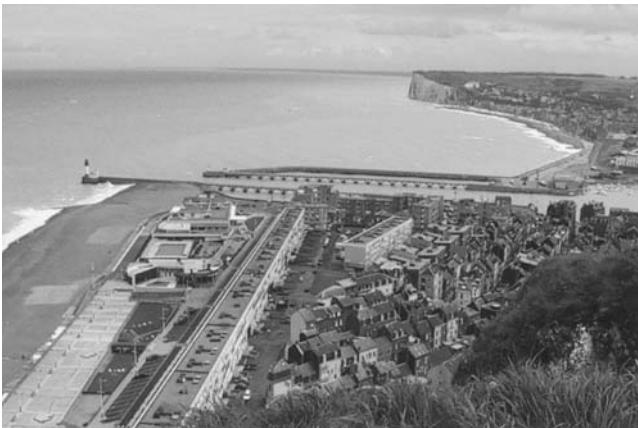
Figure B20 Beach accumulation and erosion, respectively, updrift and downdrift of a jetty in Upper Normandy, France. Erosion on this coast has been exacerbated by the stabilization of cliffs that hitherto supplied flint clasts to the beaches.
