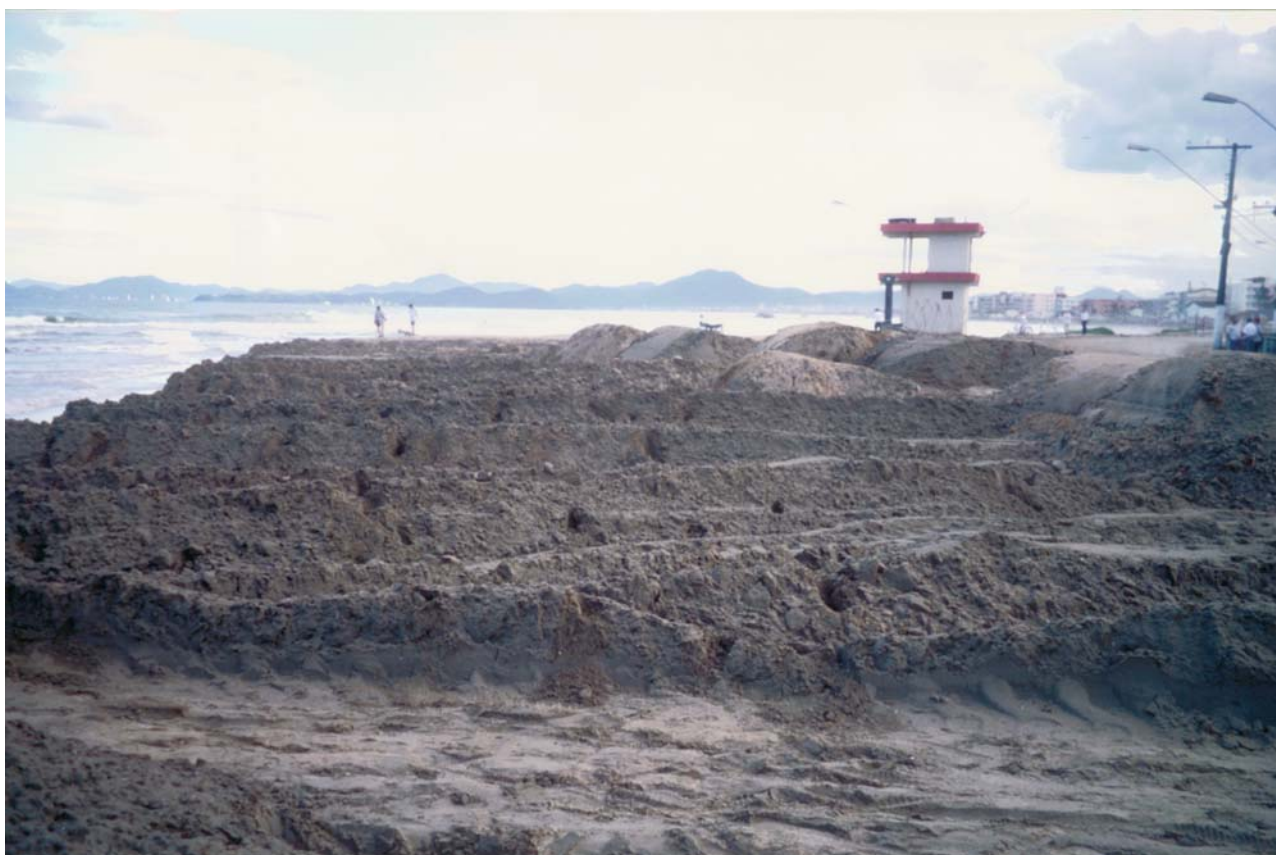
Figure B29 Emergency beach renourishment at Gravatá Beach, Santa Catarina, Brazil. A coastal highway and commercial infrastructure was threatened by beach erosion during a strong southeaster that brought heavy surf conditions to the coast during the Southern Hemisphere winter of 1999. Removal of the beach by wave and current action, undermined part of the coastal highway interrupting coastal access. Although of finer grain size than the native beach sand, emergency fill was trucked to the site for immediate shore protection.
