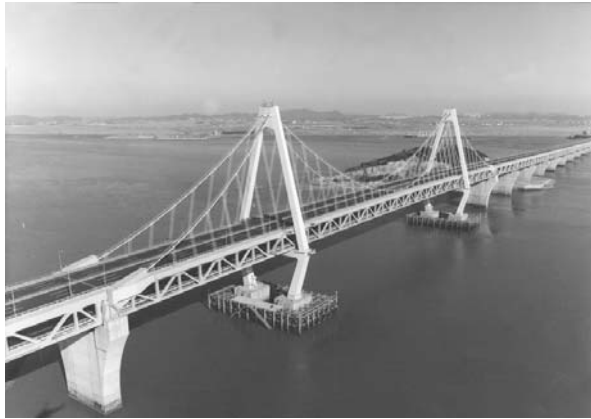
Figure 1. Overview of Yeongjong Bridge
