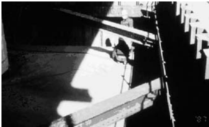
Photo 6. Direct inspection for pile damage
