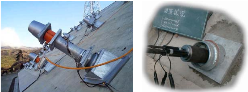
Figure 7. Intelligent ground anchor.
