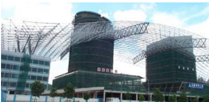
(a) The middle span of roof under constructed
