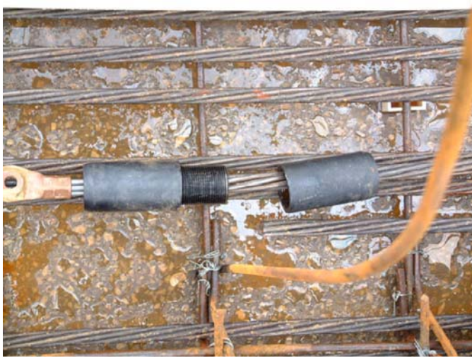
Figure 7. Connection of SMA bundle with pre-stressed steel strand
