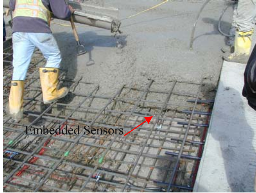
Figure 11 Embedded sensors during concrete placement
