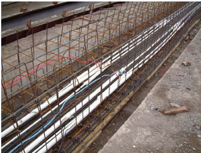
Figure 8. Photograph of SMA bundles in framework of steel reinforcement
