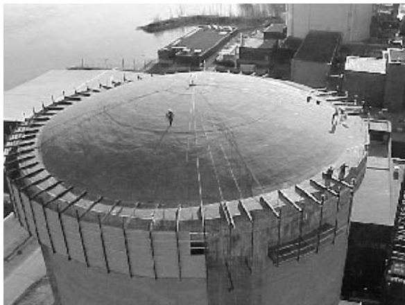
Figure 3. Gentilly Nuclear Secondary Containment Structure
