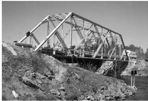
Figure 5. Truss bridge being tested to failure
