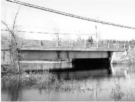
Figure 2. View of the Sainte-Émélie Bridge
