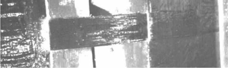
Figure 10. Rupture of restrainer
