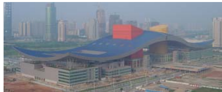
(b) The building after constructed
