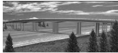
Figure 10 Dongying Yellow River Bridge in Shandong (2003, over 1800 FBGs used)
