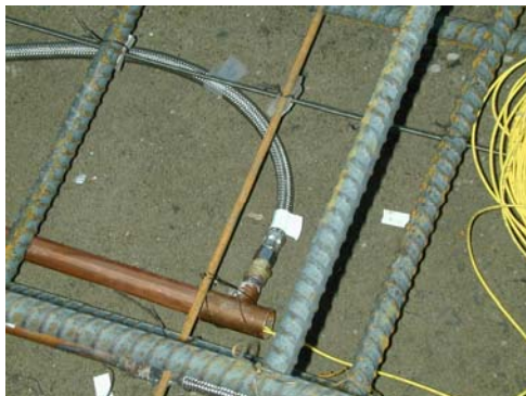
Figure 13 Details of sensor lead out route through specially designed Brass conduits
