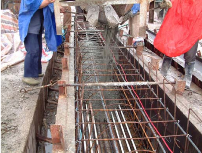
Figure 11. Photograph of depositing concrete
