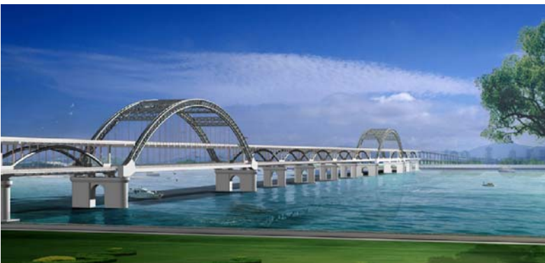
Fig. 2 Visual painting of Qianjiang No. 4 Bridge
