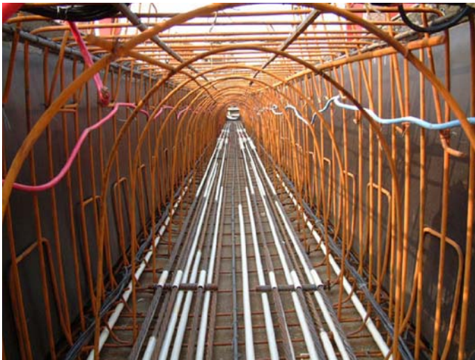
Figure 10. Photograph of framework of steel reinforcement with stretched SMA bundles
