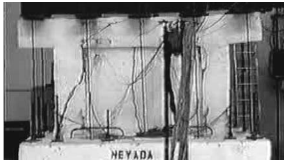
Figure 6. Opening of shear crack in the left column
