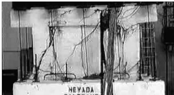
Figure 7. Start of shear/compression failure in top of right column
