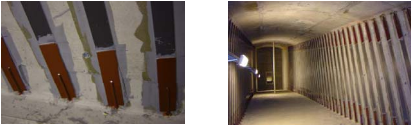
Figure 2 a) Anchor system for the CFRP laminates. The anchorages are bonded with an epoxy adhesive in pre-drilled holes in the flanges, b) Final result after strengthening
