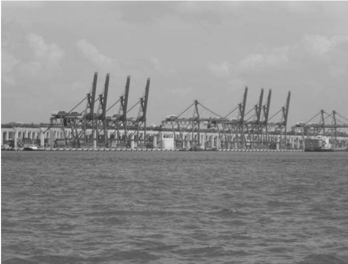
Figure 2. Part of the container port along the southwest coast. The original coastal habitat is buried by coastal reclamation and replaced by concrete structures.
