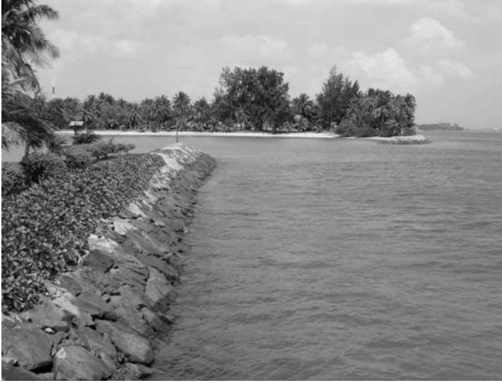
Figure 4. Reef-flats of some of the southern offshore island were transformed to sand-bottom swimming lagoons. They are protected by retaining seawalls.
