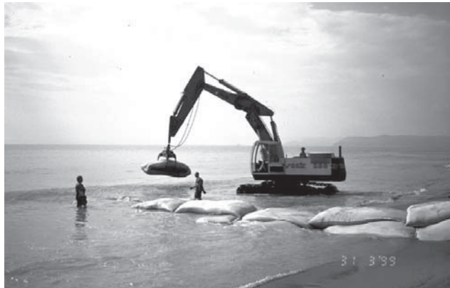
Figure 11: Submerged groins construction at Marina di Ronchi (Tuscany, Italy)
