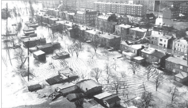
Figure 11: Non-Stress-Resistant Infrastructures behind Coastline
