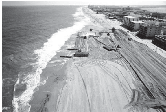
Figure 16: Beach Nourishment of Eroding Coast
