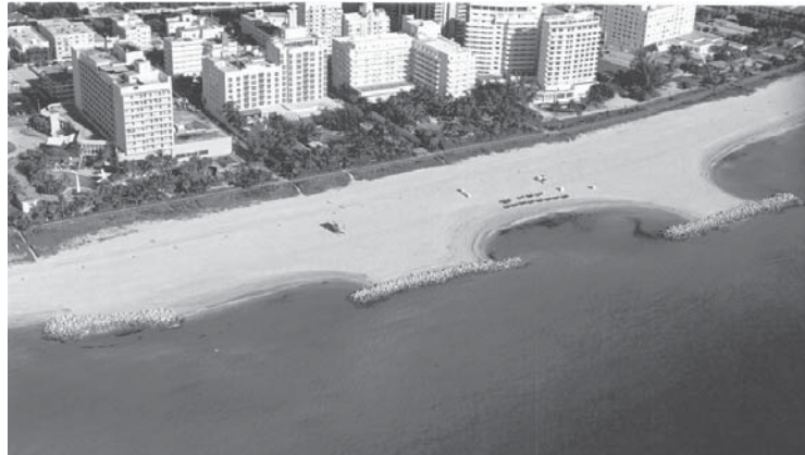
Figure 12: Headland structures, Miami Beach, Florida
