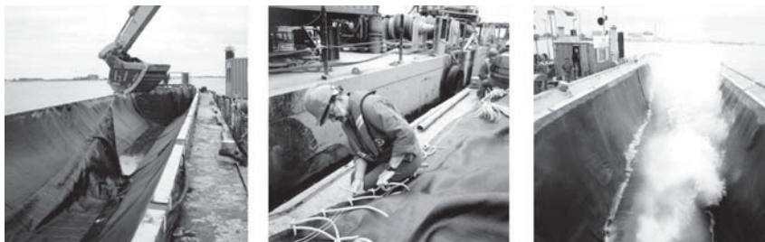
Figure 9: Placing a Geocontainer (Photos Rijkswaterstaat, DWW)
