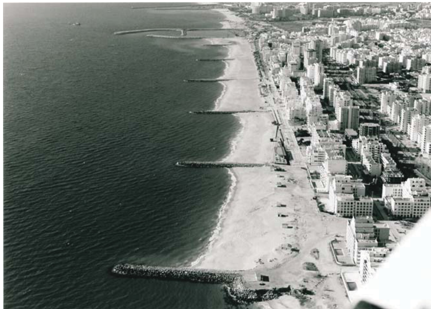
Figure 2: Aerial view of coastal structures in front of Quarteira
