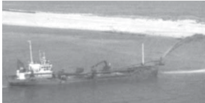
Figure 6: Artificial nourishment of Danish west coast with rainbow method (Viking R dredger)
