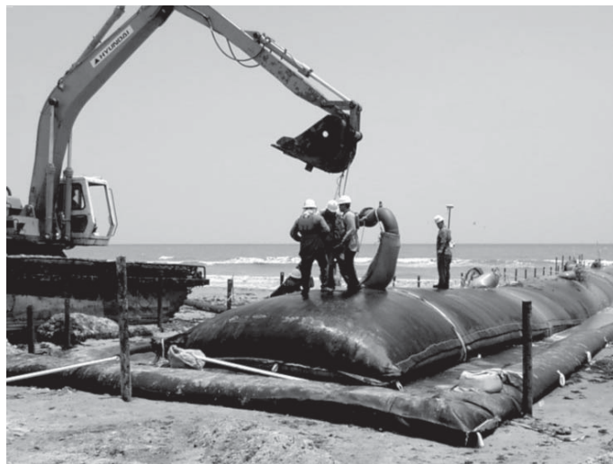
Figure 7: Geotextile tube groin construction, Jefferson County, Texas
