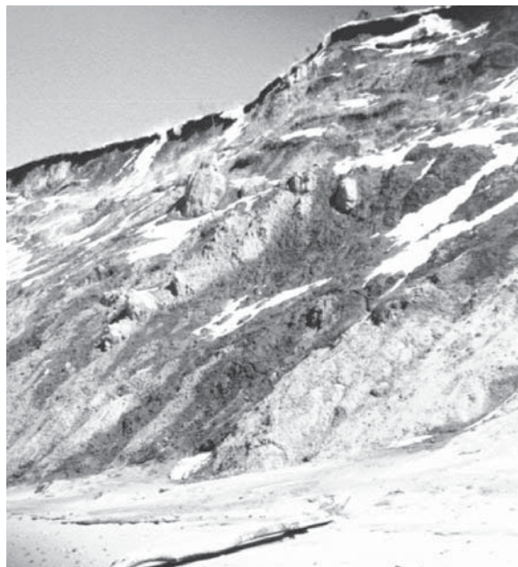
Figure 9: Frozen perched groundwater seeps on bluff face, Allegan County Michigan
