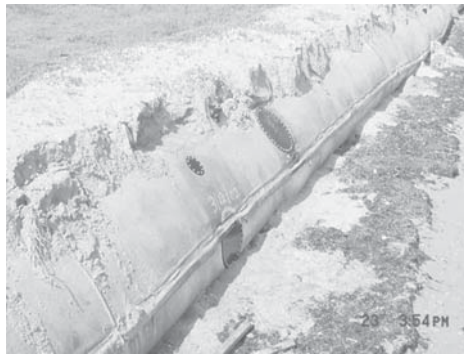
Figure 13: HDPE repair plates for a Geotube (Heilman & Hauske, 2003)
