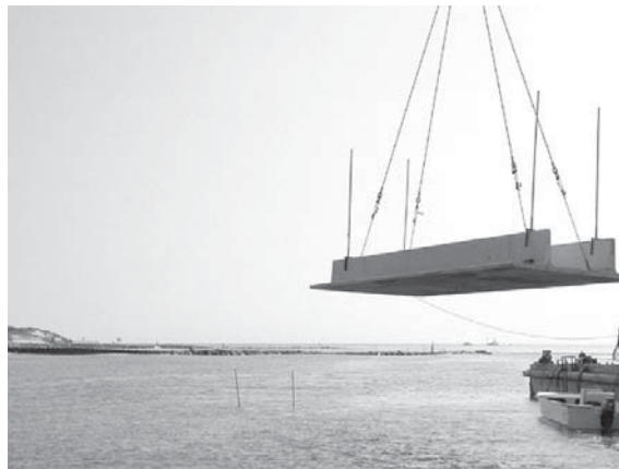
Figure 4: Placement of Double-T sill unit, Cape May Point, New Jersey
