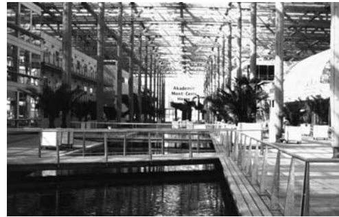
Figure A40 The glazed superstructure over the office space of Moncenis in Essen moderates the northern German climate to be more like Tuscany.
