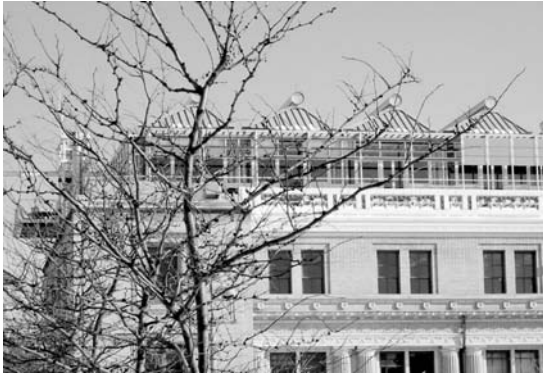
Figure A39 Atop a 100-year-old building, the dynamic enclosure of the Intelligent Workplace™ at Carnegie Mellon University uses sunlight and natural ventilation to achieve an 80% reduction in heating, cooling and lighting loads of typical office buildings.
